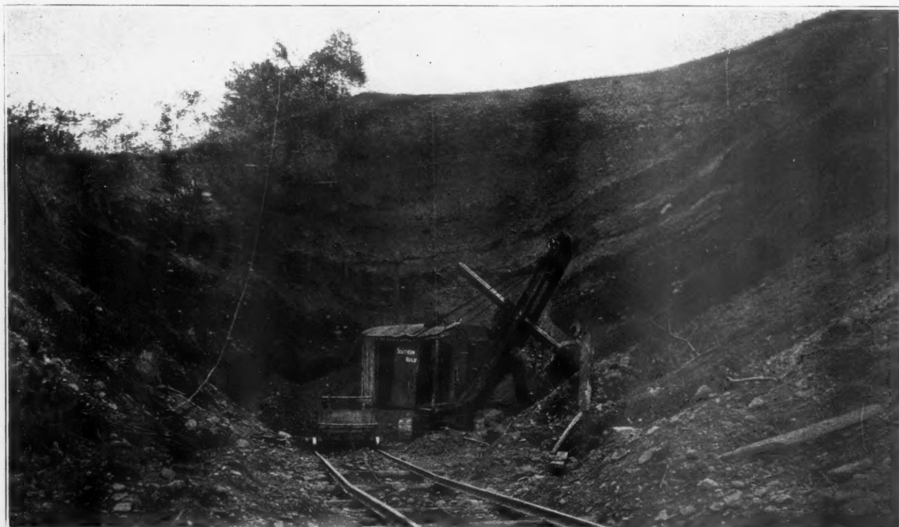
Electric Shovel Loading Dump Car in Pit
